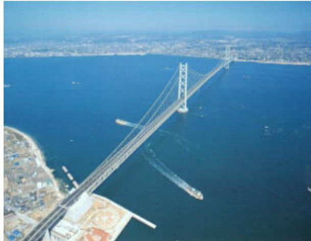
**Figure 3: Akashi Kaikyo Bridge (3-span 2-hinged truss-stiffened suspension bridge)**
