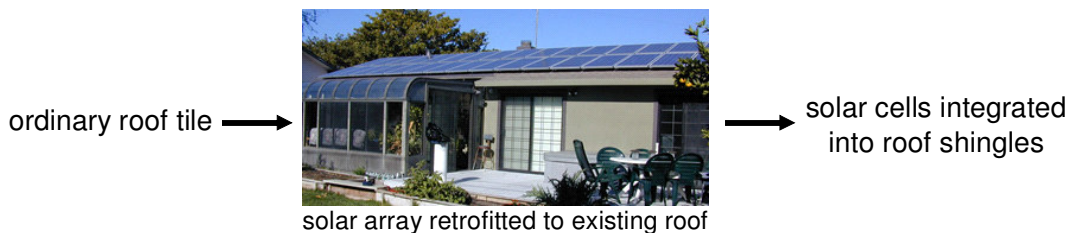
Figure 2: Typical Solar Panel Added Onto An Existing Roof
